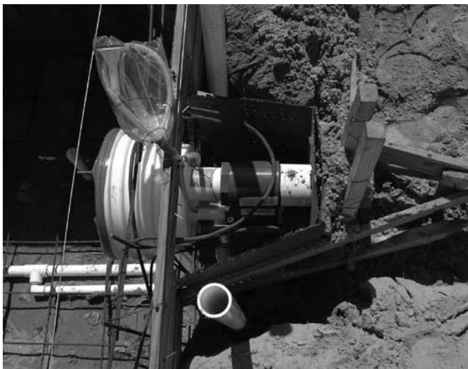
Fig. 7 Setting the BADUJET housing into reinforced steel
