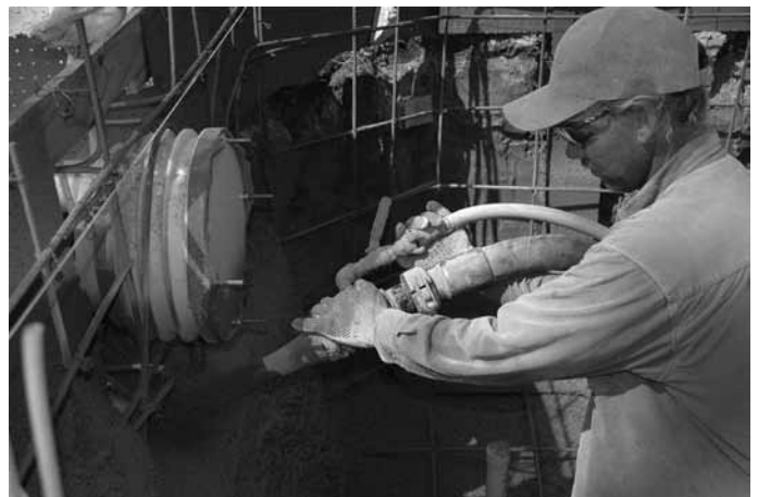
Fig. 8 BADUJET Ready for Guniting
