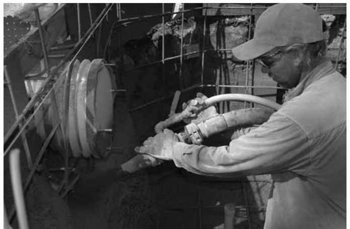
Fig. 8 BADUJET Ready for Guniting
