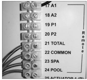
Fig. 10: Heater Wiring Block — Analog Heaters
