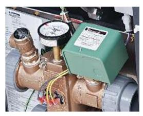
Flow switch, PRV and T&P gauge-standard
