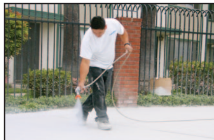
SECOND COAT (FULL STRENGTH COAT) CAN BE APPLIED BY AIRLESS SPRAYER OR ROLLER.
