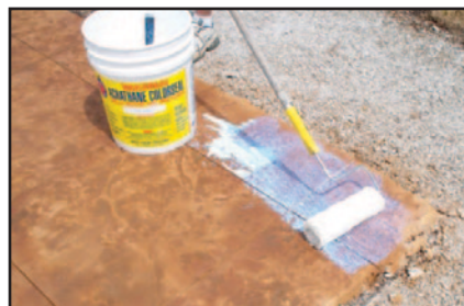
CLEARSEAL GOES ON WHITE AND DRIES TO A CLEAR FILM IN MINUTES. CAN BE ROLLED OR SPRAYED.
