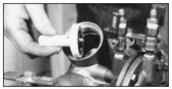
The line should be flushed clean of debris before installation of the assembly. To flush the line after installation of the assembly, slowly close the inlet shut-off valve, remove the covers and internal assemblies of both check valves and open the inlet shut-off valve to allow sufficient flow of water through the assembly to clear all sand, debris, etc. from the line. If debris in the water continues to cause fouling, a strainer may be installed upstream of the assembly.
