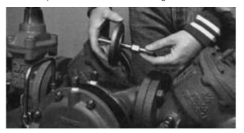
NOTE: On older Model 825 valves, the disc holder is sealed to the stem with a sealant. If the seal is broken, the stem and holder must be cleaned and new sealant applied. Newer valves, Models 825D and 825YD, use an o-ring so a sealant is not required.
