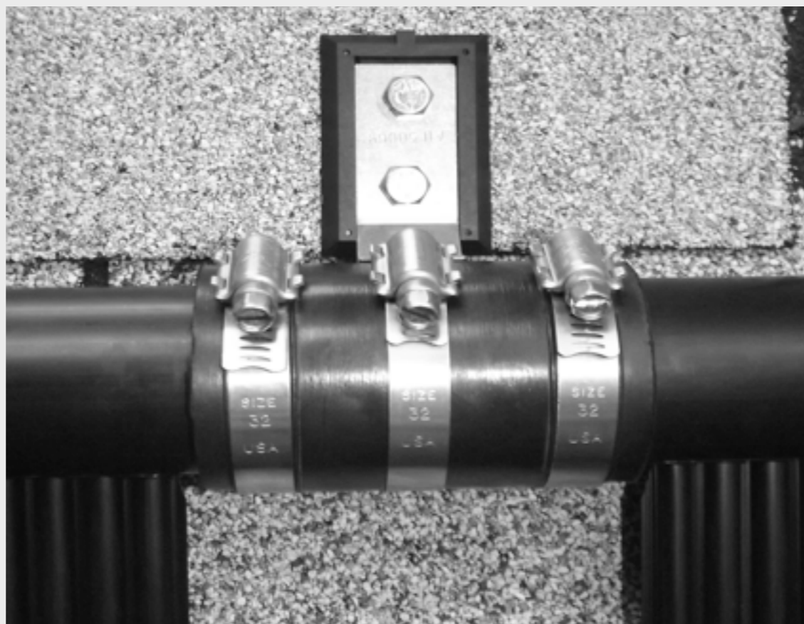
FIGURE 5 Installed Outlet Header Bracket with Hose
