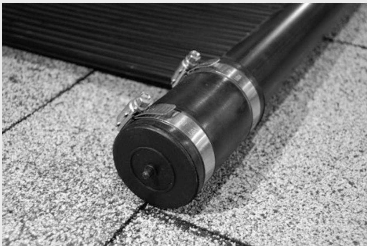
FIGURE 11 Installed End Cap
