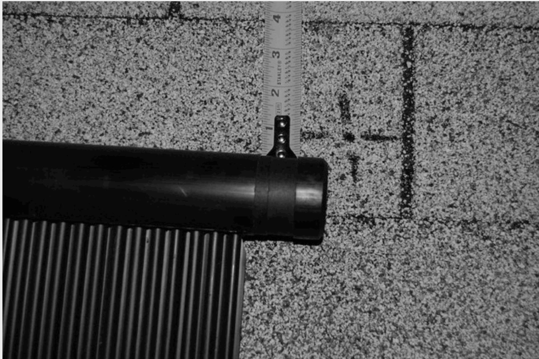
FIGURE 3 Outlet Header Bracket Location
