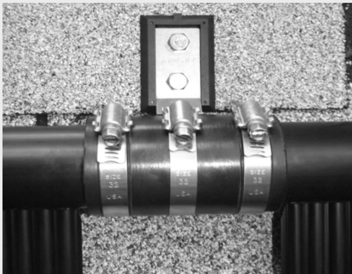
FIGURE 5 Installed Outlet Header Bracket with Hose
