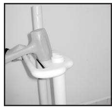
**Step 5:** Install towel rack/cup holder over the handrail posts with the towel rack to the outside of step, tap in place using the rubber mallet. Towel rack/cup holder may be positioned anywhere on the post.
