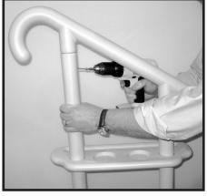
Step 7: Secure handrails using 1- # 10 x 1%" screw into each post at pre-marked locations.
