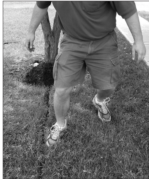
In turf, the trench is easily closed by gently pushing in from both sides.
