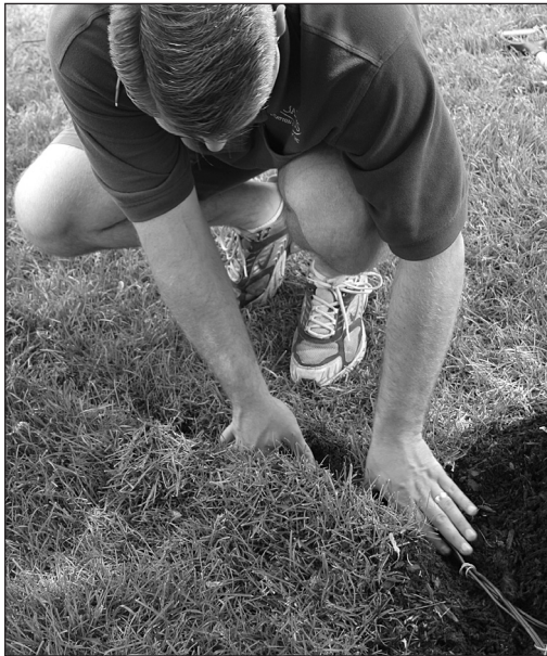
Wires are pushed firmly into the trench.
