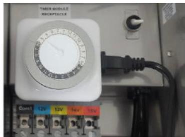
Follow the instructions for the timer to set the clock to on and off times or manually turn on/off your system.
