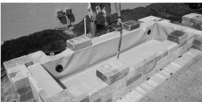
As you are filling the basin with water, continue smoothing out the wrinkles from basin as you go, making sure to tuck the basin corners tightly into place. During this process, the basin can be filled to the bottom of the bulkhead opening. For best results, temporarily install a 1 ½" plug in the bulkhead in order to fill the basin to within a couple inches of the top of the basin (Figure 4).
